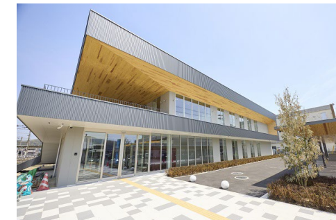
Nine facilities in the PPP business commenced management and operation
